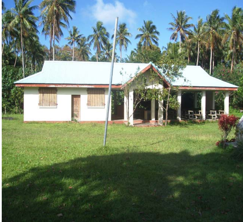
[Court House: Morua, Tongoa Island]
